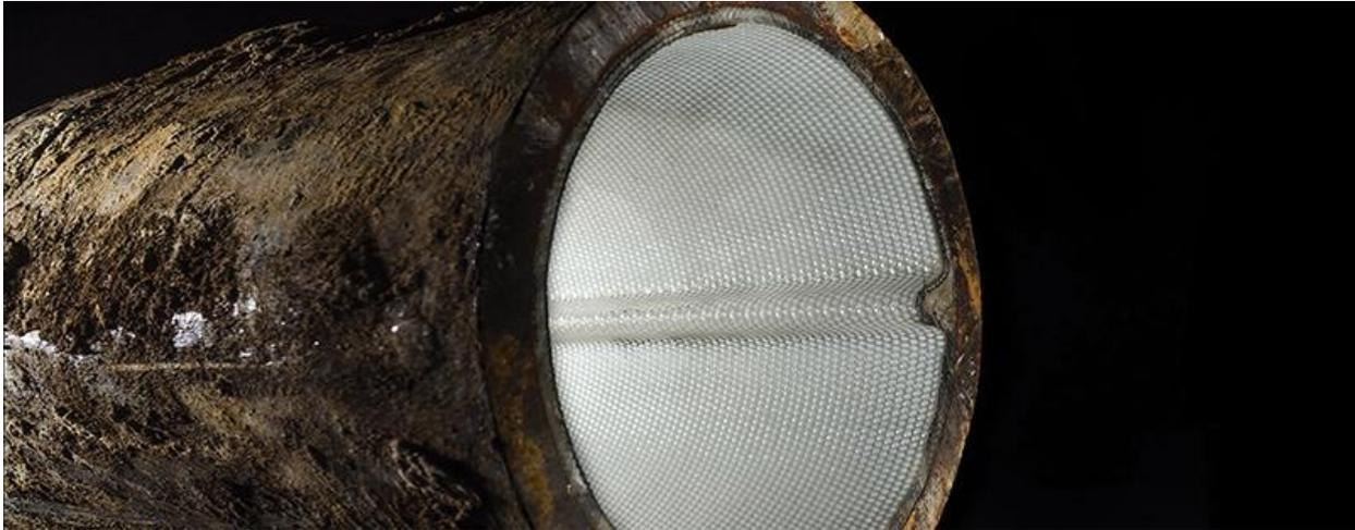
Over the years, the City of Toronto's Watermain Rehabilitation Program has been delivering cured-in-place-pipe (CIPP) watermain structural lining and cathodic protection of existing watermains. (WSP)
