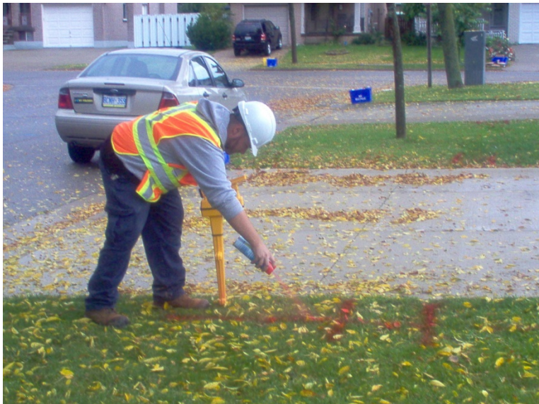
A worker sprays a lawn to mark the location of buried infrastructure.
